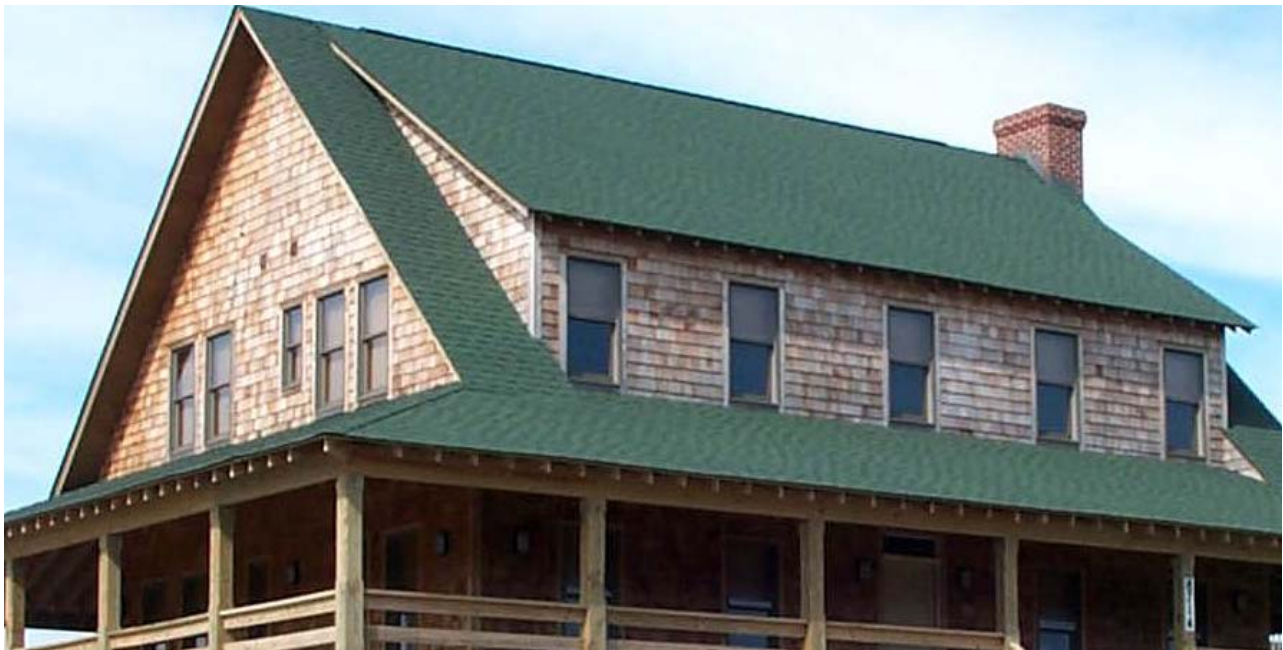
Wood Shingle Siding
